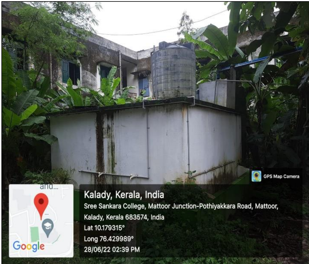
Rain Water Harvesting System at Sree Sankara college, Kalady
