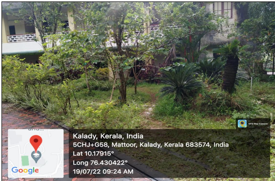
Waste Water Recycling in the campus for irrigation
