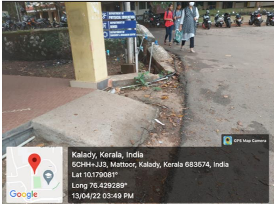
Ramps constructed to assist Divyangjan Students
