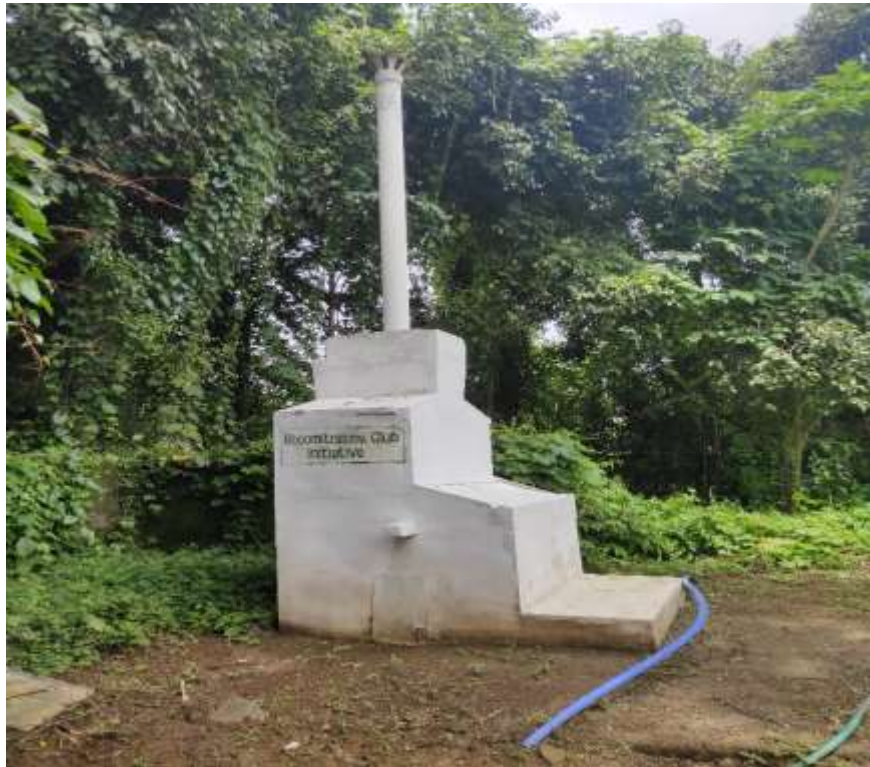
Figure 3 OPEN TYPE INCINERATOR
