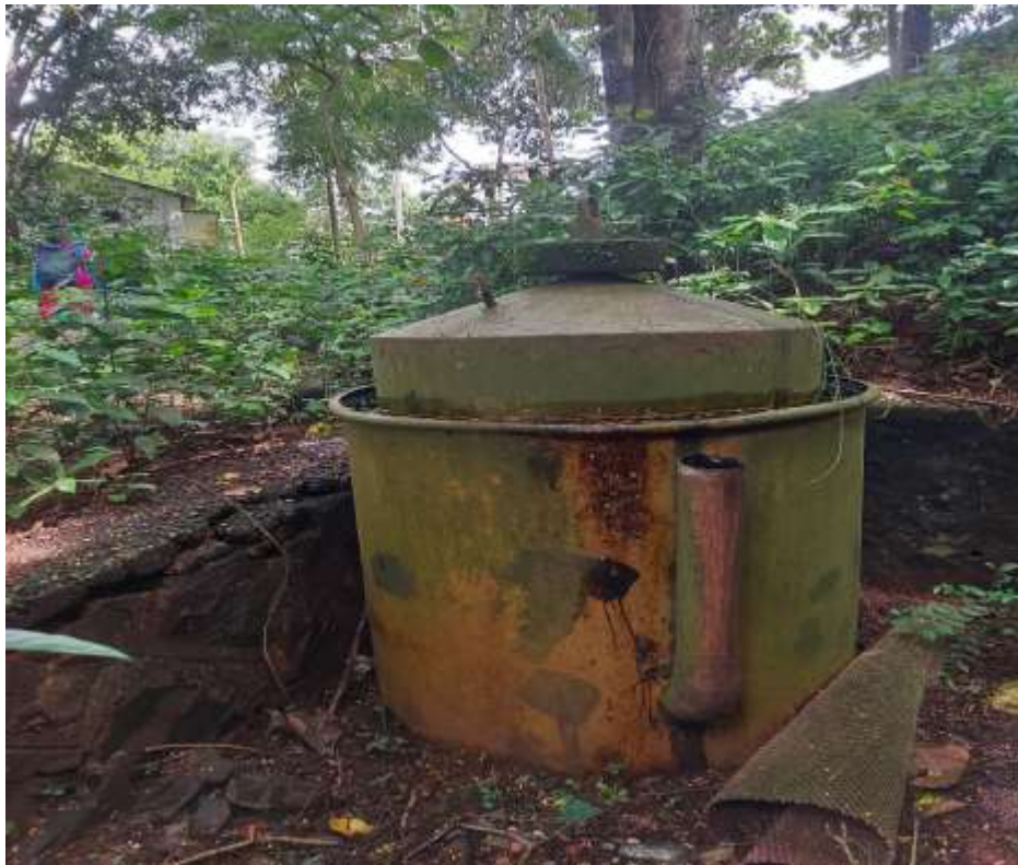
figure 2 FRP BIO GAS PLANT
