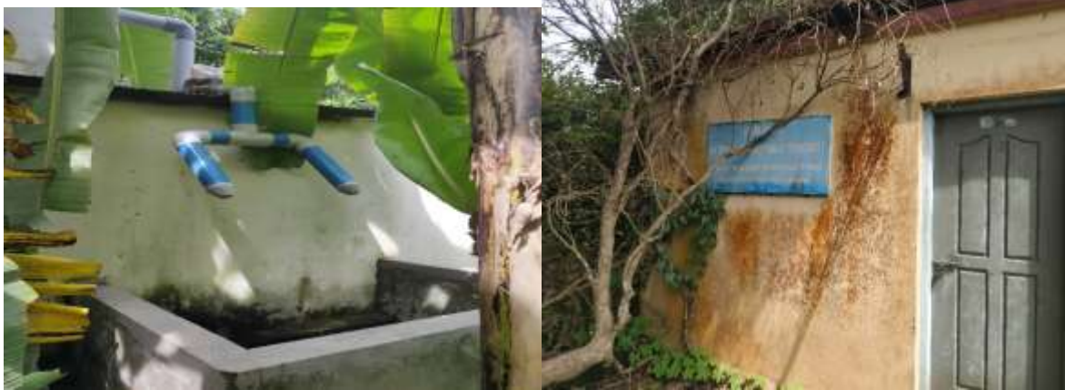
Figure 10RAIN WATER COLLECETION
